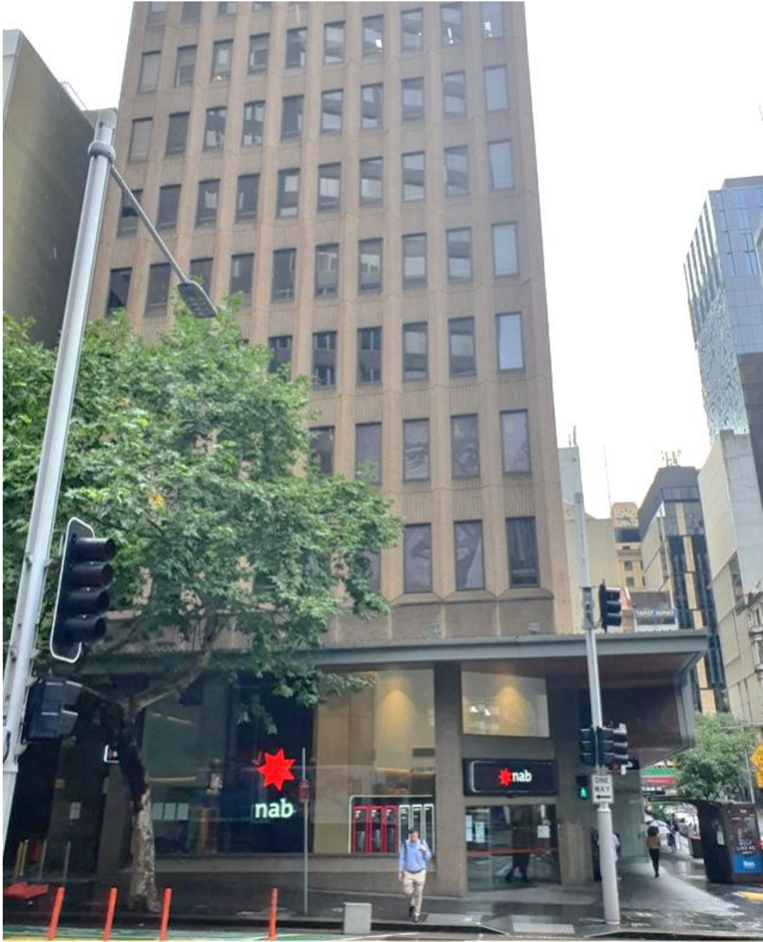
Figure 2-23 Existing commercial building at 20-25 Pitt Street
