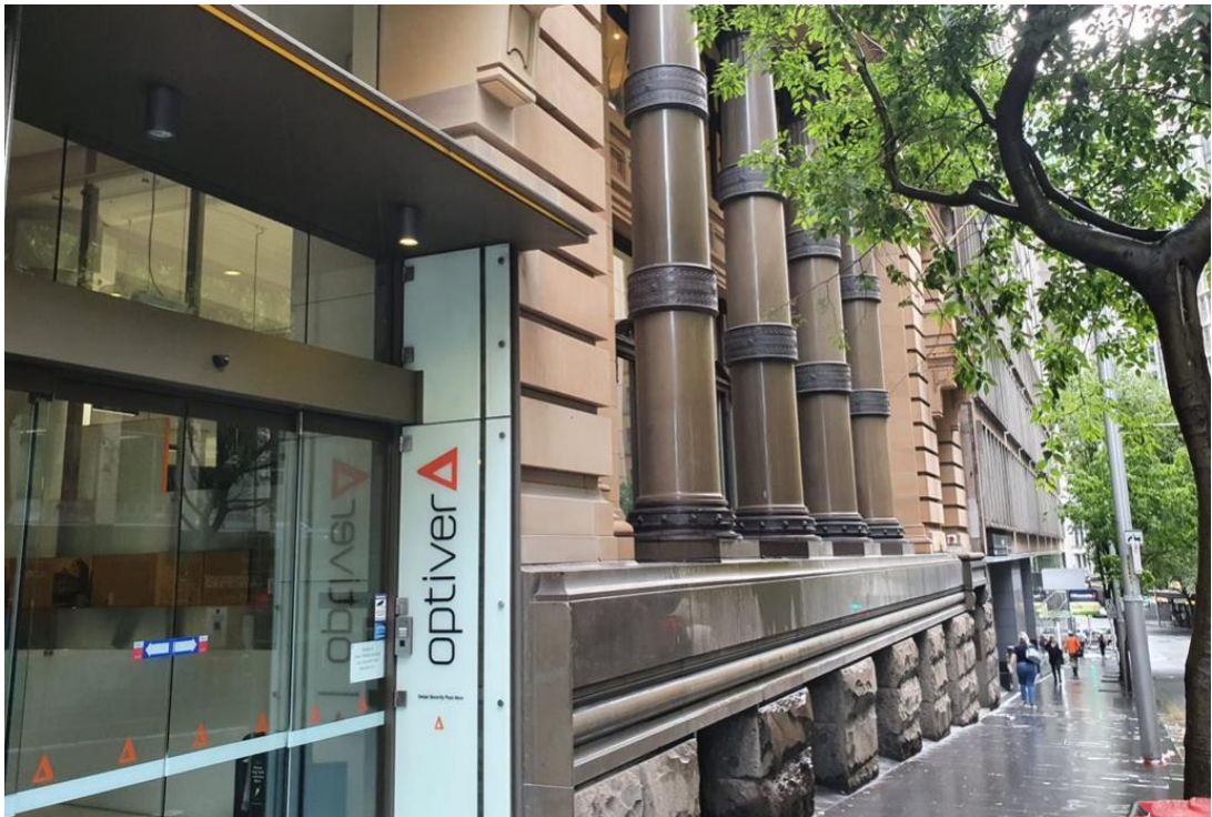
Figure 2-20 Heritage listed commercial building at 39 Hunter Street
