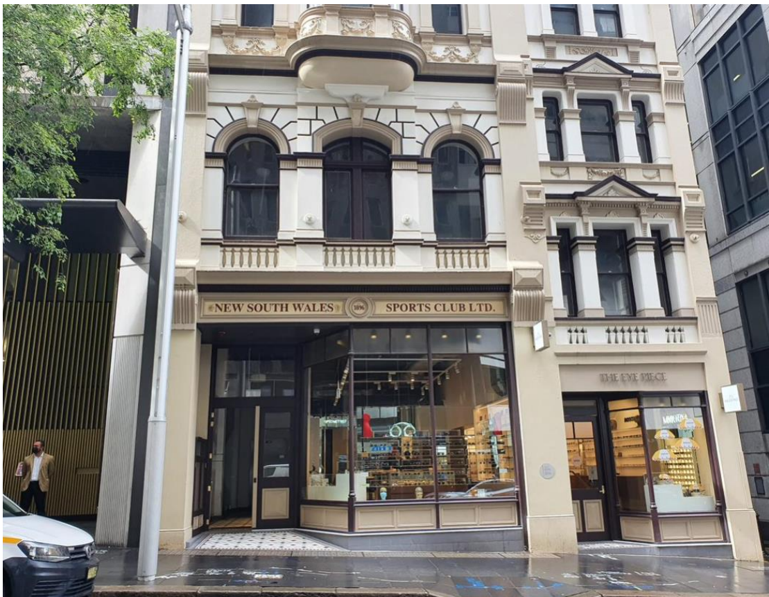
Figure 2-22 Commercial buildings on the opposite side of Hunter Street
