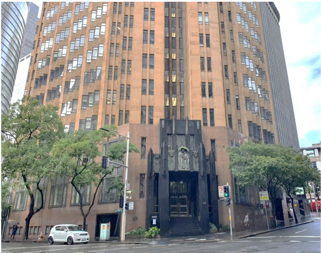
Figure 2-18 Heritage listed City Mutual Life Assurance Building at 10 Bligh Street
