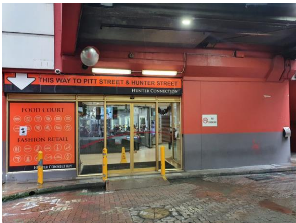
Figure 2-12 De Mestre Place with overpass above (5010 De Mestre Place)
