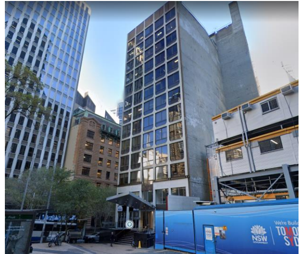
Figure 2-8 Building at 48 Hunter Street, facing south-west
