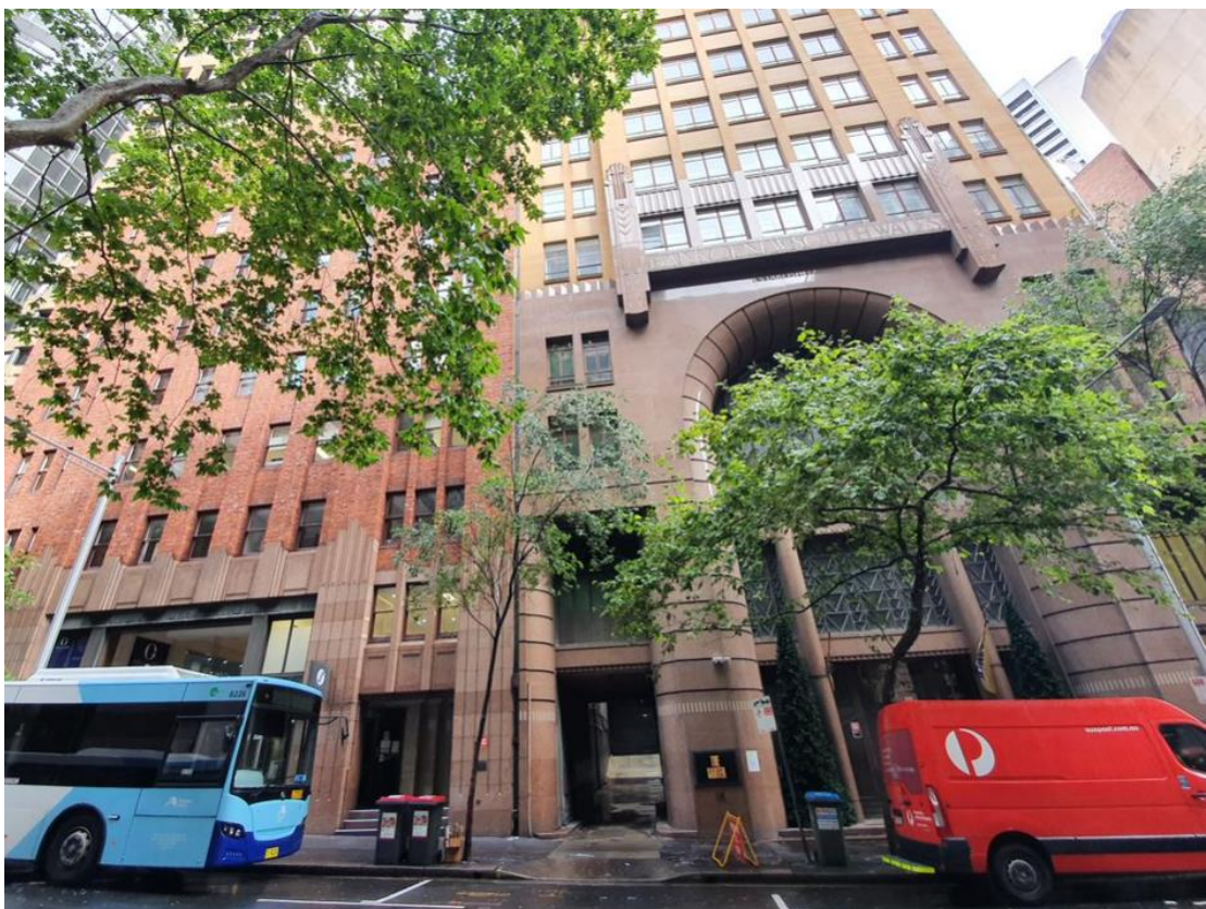
Figure 2-15 Existing heritage listed buildings at 12-14 and 16 O'Connell Street
